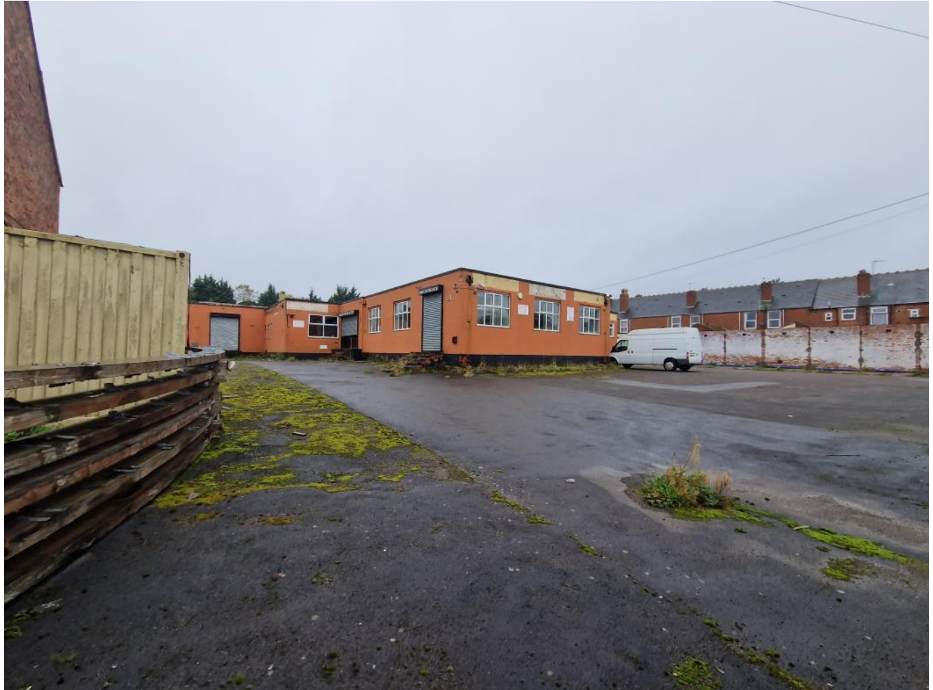
Existing building on site
