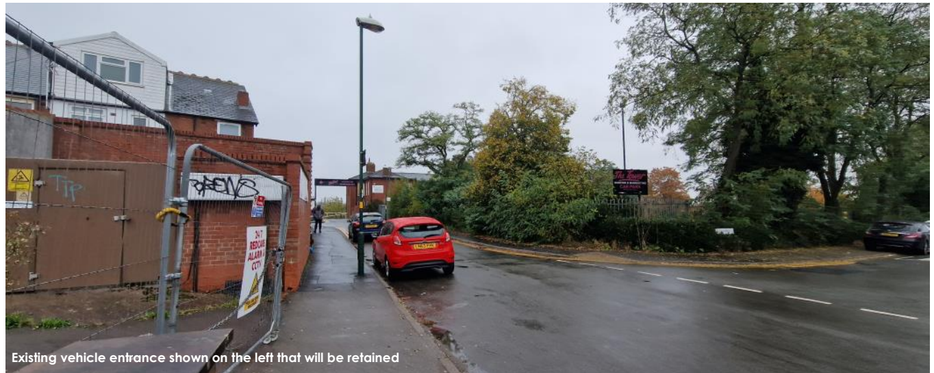
An existing pedestrian opening that is proposed to be widened for a second vehicle entrance
