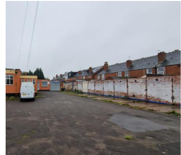
View of west boundary showing a 2.4m tall brick wall
