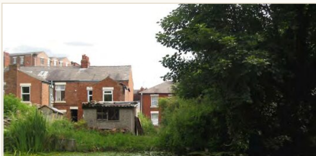
THE SITE FROM THE CANAL SIDE
