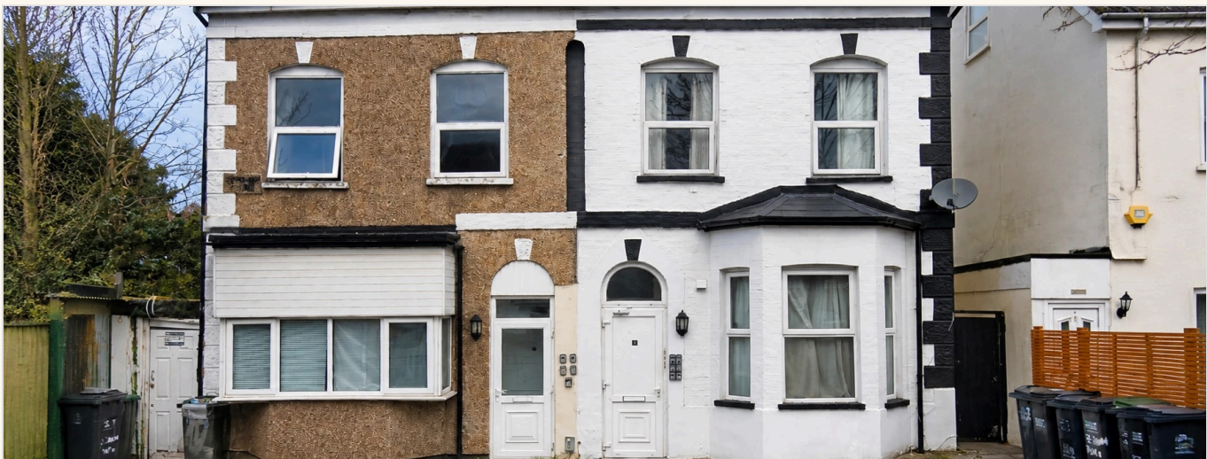
3 Beulah Road – front elevation and paved frontage.
