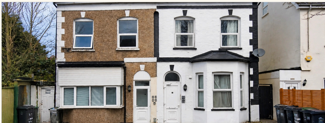
5 Beulah Road is the white-fronted house on the right. The left-hand house, No. 3, is offered separately as Lot 38.
